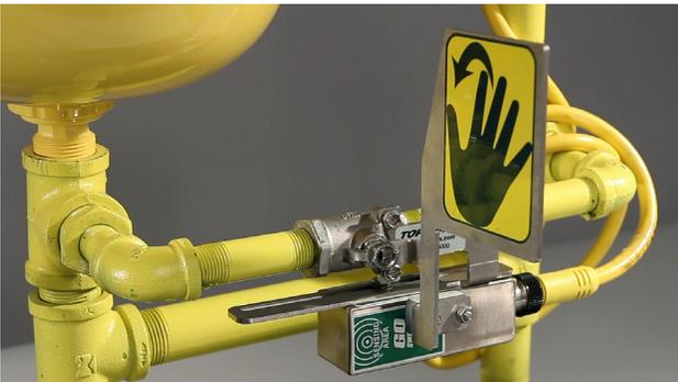
**Figure 20. Eye Wash in Activated Position**
