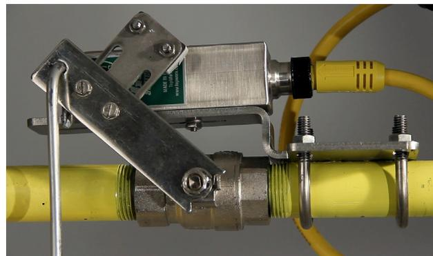
**Figure 18. Safety Shower Valve in Activated Position**
